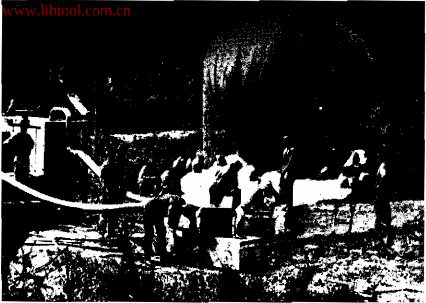
Civil War balloon filling from hydrogen-generating equipment on left.
