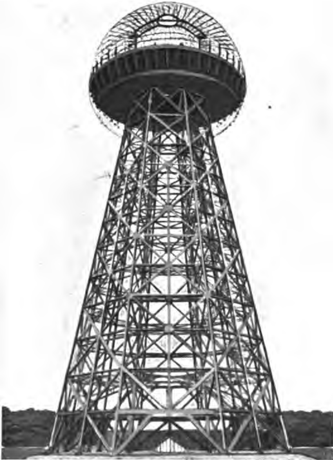
FIG. 125.—MR TESLA'S TRANSMITTING STATION ON LONG ISLAND.
