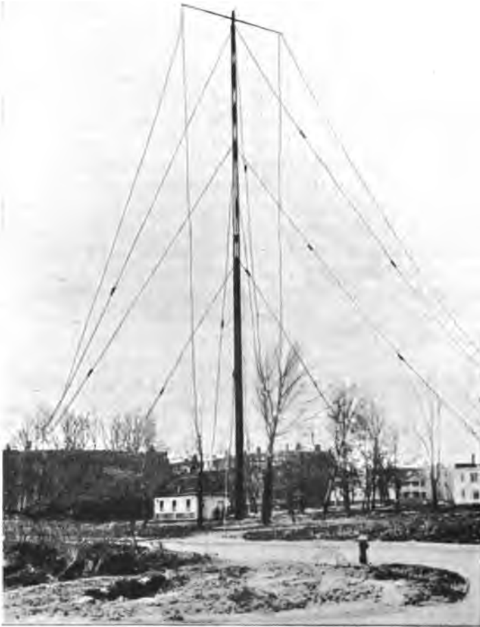
FIG. 101.—BOSTON STATION OF THE DE FOREST WIRELESS TELEGRAPH COMPANY.
