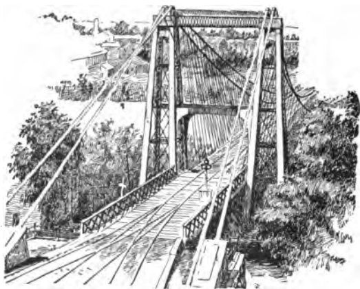
The New Iron Towers of the Niagara Bridge.
