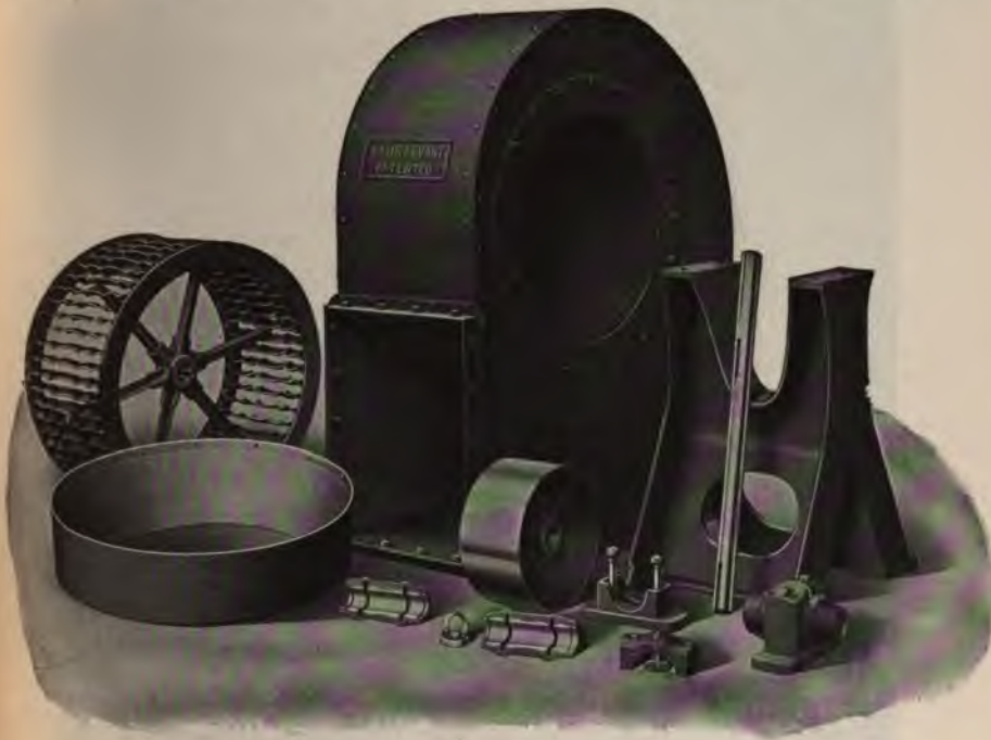
FIG. 13.—Sturtevant Multivane Fan. Details of Casing, Runner, Pedestal, and Bearings.
