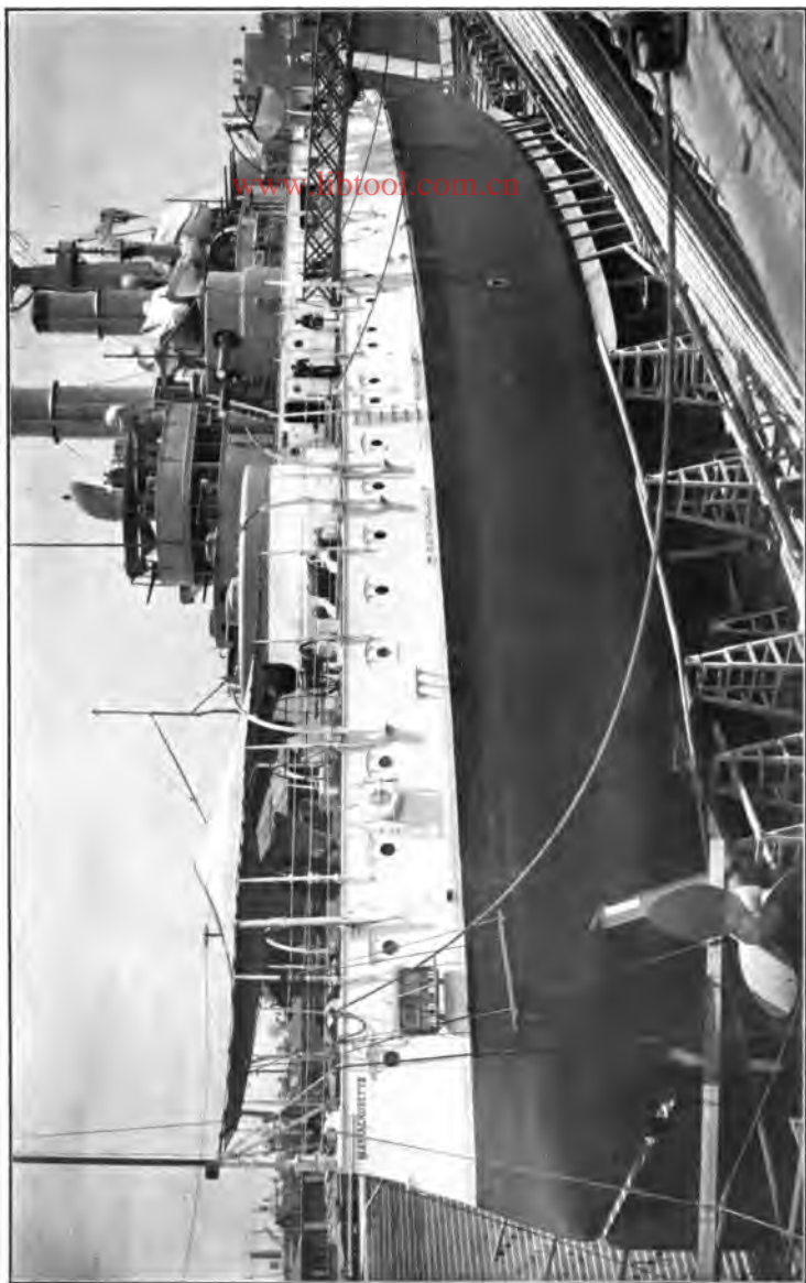
HOW A BATTLESHIP IS DOCKED. The Massachusetts in dry-dock. This ship is about ready to be undocked. Copyright, 1906, by Enrique Muller.
