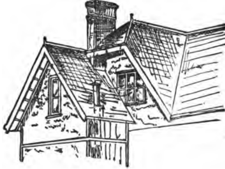
FIG. 30.—A soil pipe terminating near attic window.
