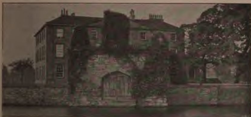
WALTON HALL. ( View showing Water Gate. )
